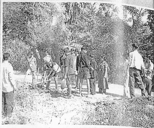
Assisting the villagers in Road repairs NSS Camp
